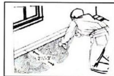
Use Tapping Block if necessary to fit planks snug together at side and butt ends. Clean any adhesive off the surface before it cures using clean terry cloth towels and mineral spirits.
